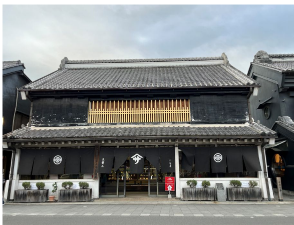
Figure 3: The Ōsawa residence, Kawagoe. Photo: Toyozawa Chikako
